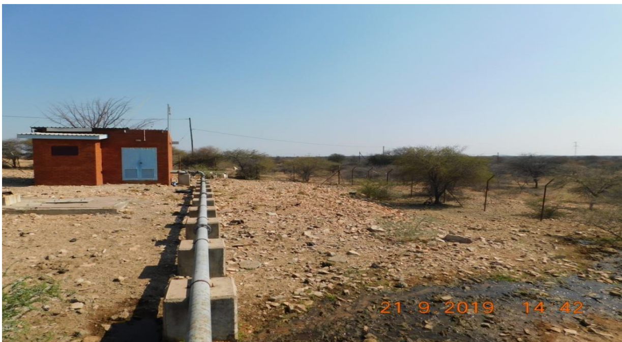
Existing Pump Station
