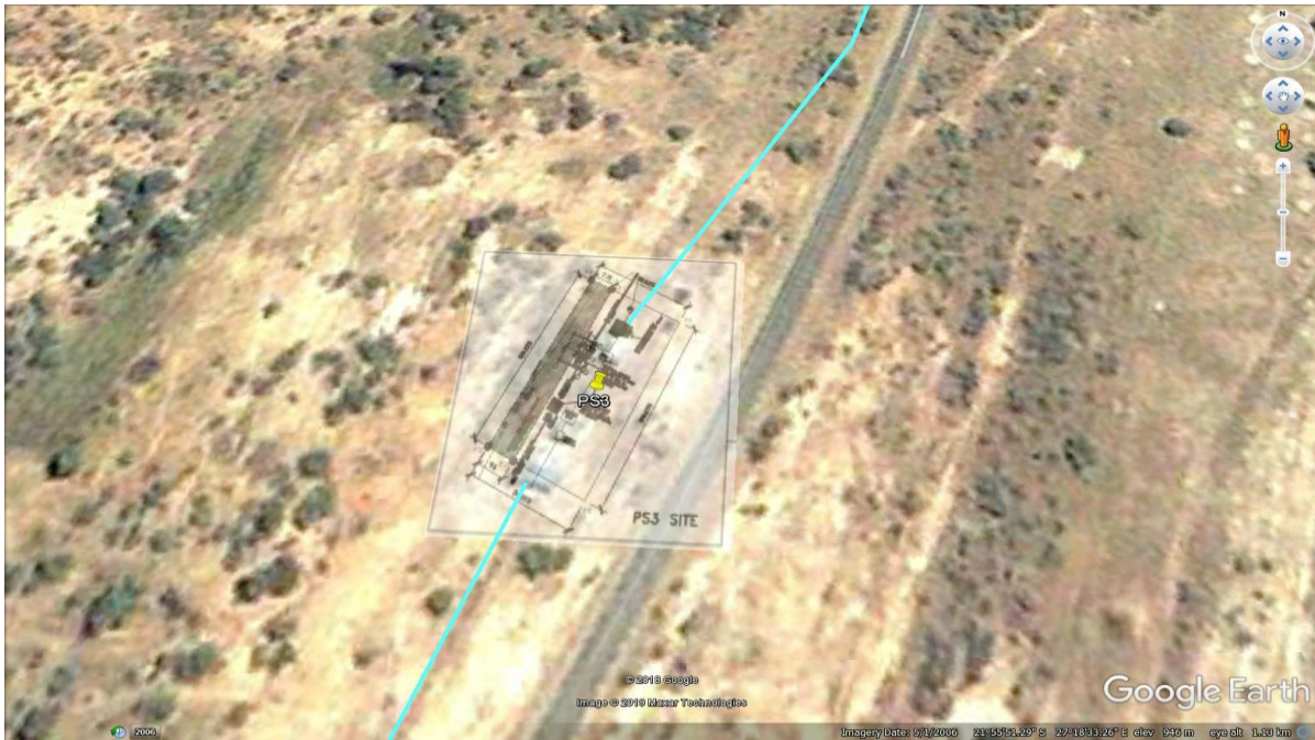
Overlay Aerial Photo Showing Existing and Extension Sites.
